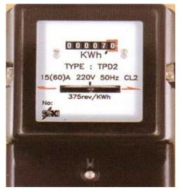
Some meters have special counters whose index should be multiplied by 10. For more detail don't hesitate to ask any of EDL's collectors to help you understand your meter better.
